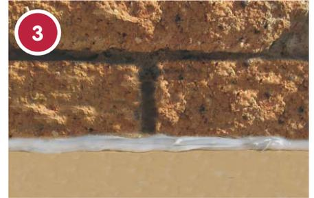
To allow for movement a 10mm bead of flexible silicone must be applied into all internal corners and interfaces prior to the TAL Sureproof application.
