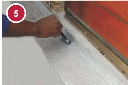
Apply a coat of TAL Sureproof by short hair enamel paint roller or brush to the interfaces. Immediately bed a 200mm wide strip of TAL Sureproof Membrane into the wet TAL Sureproof, with the membrane extended 100mm on either side of the interface. The membrane must be pushed into the corners. Apply a heavy topcoat of TAL Sureproof over the membrane to saturate the membrane before the first coat dries.
