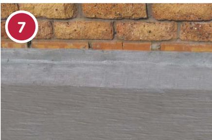
It is essential to ensure that the main TAL Sureproof application overlaps the corner joints/interfaces, i.e. the interface application must be completely covered by the main area application.
