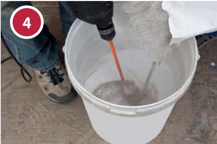
The two parts are mechanically mixed together by adding the powder to the liquid, and mixing until a creamy, lump-free consistency is obtained. Let the mix stand for 3-5 minutes before stirring again.
