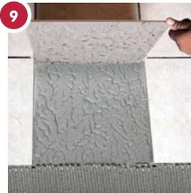
9 Lift the occasional tile to check for full coverage of adhesive on the back of the tile. No voids should occur underneath the tiles.
