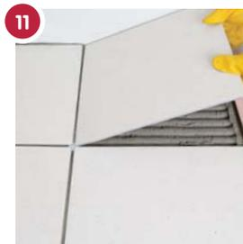
11 Measure and cut each tile to fill edges leaving room for the tile spacers. Butter the back of the tile with adhesive, place the cut edge towards the wall and bed firmly into place using a rubber mallet.
