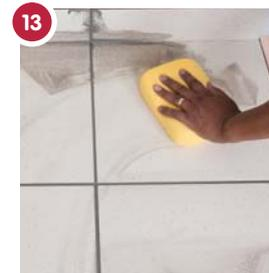
13 Remove the excess grout with a sponge. Allow the grout to dry and then polish with a dry cloth.
