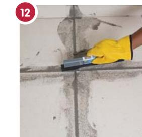
12 Allow the adhesive to dry before grouting. Use TAL Wall and Floor Grout or TAL Quarry Grout available in a variety of colours. Work grout well into joints with a rubber squeegee.
