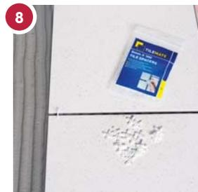
8 Use tile spacers to create uniform spacing. Remove before grouting. Never butt ceramic tiles hard up against each other.
