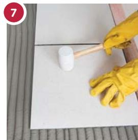
7 Use dry tiles. Butter the back of heavily ribbed tiles. Bed the tiles firmly into the adhesive using a rubber mallet.
