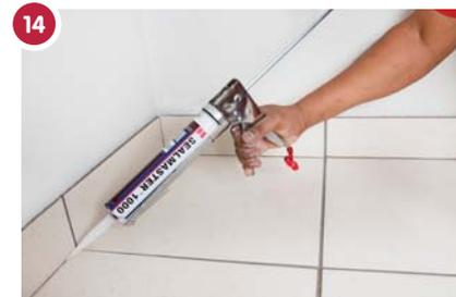
14 Provide movement joints in all corners. In large tiled areas keep these approximately 5m apart internally and 3m apart externally. Rake out joints and leave ungrouted. Fill with TAL Goldstar Sealmaster 1000 polyurathene joint sealant.
