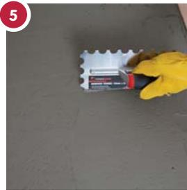
5 Start at the centre of the room. Use the appropriate TAL adhesive, like TAL Goldstar 6, and with the straight edge of a floor trowel, spread the adhesive onto the floor.
