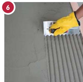
6 In a horizontal direction, notch the adhesive with the floor trowel or floor applicator. Do not spread more adhesive than can be tiled onto in approximately 15 minutes.
