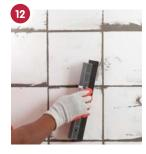
Allow adhesive to dry before grouting. Use TAL Wall and Floor Grout, available in a variety of colours. Work grout well into joints with a rubber squeegee.
