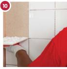
Measure and cut each tile required to fill in corners and bottom row, leaving room for tile spacers. Butter the back of the tile with adhesive, place cut edge into the corner and press firmly into place.
