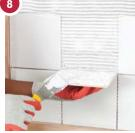
Bed the tiles in firmly using a rubber mallet. Remove the occasional tile to check that good contact with the adhesive is being made.
