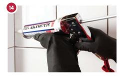
Provide movement joints in all horizontal and vertical corners. In large areas keep these approximately 5m apart. Rake out joints and leave ungrouted. Fill with TAL Goldstar Sealmaster 1000 polyurathene joint sealant.
