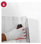
In a horizontal direction, notch the adhesive with the notched wall trowel or wall applicator. Do not spread more adhesive than can be tiled onto in approximately 15 minutes.
