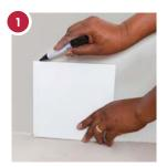
Find the lowest point on the floor line and mark the wall one tile high from the floor at this point.
