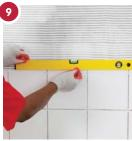
Check tiling regularly with a spirit level to ensure that horziontal fixing is being maintained.
