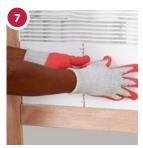
Using dry tiles, begin in the corner of the battens placing tiles horizontally. Tile spacers ensure even joints between tiles. Remove before grouting. Leave cut tiles until last.
