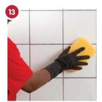
Remove the excess grout with a sponge. Allow the grout to dry and then polish with a dry cloth.
