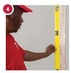
Nail a vertical batten to the wall so that the inside edge of the batten coincides with the mark for the first tile. Check with a spirit level to ensure that the batten is perfectly vertical.
