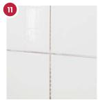
After the adhesive has set, remove horizontal and vertical battens.
