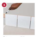
Set out a row of tiles across the wall over the batten and adjust so that equal cuts at least half a tile wide will be made in each corner. Mark the batten where the first tile will be placed.
