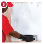
Use the appropriate TAL tile adhesive, like TAL Flex, and commencing in this corner, spread the adhesive onto the wall with the straight edge of a notched wall trowel or wall applicator.
