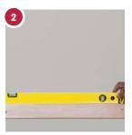
Nail a batten with a straight edge to the wall so that the top edge of the batten coincides with the mark. Ensure that the batten is horizontal, by using a spirit level.
