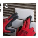
Tile the shower with a quick or rapid setting adhesive using TAL BOND as a total water replacement. Then use TAL grout mixed with TAL BOND to finish the installation
