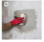
Apply the **second coat** in a horizontal direction to the first coat to ensure complete coverage
