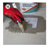
Upstairs showers only: Use a reinforcing membrane (200mm wide) in internal corners, interfaces, around tap and rose plumbing fittings as well as drains
