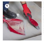
Ensure the surface is integrally sound, clean and free from any contamination, such as dust, dirt, waxes, bituminous compounds and organic or fungal growth
