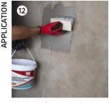
Apply the **first coat** to the clean, dry surface with a block brush in a vertical direction.
