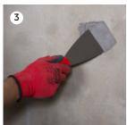
Fill any holes or surface defects with a suitable quick-setting repair compound
