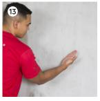
Check that the **first coat** is touch dry before applying the second coat. (1-2 hours)
